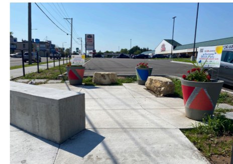
Parking Lot Renovation
