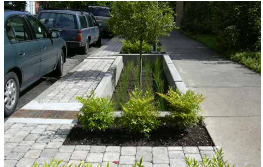
Examples of infiltration and flow-through planters
