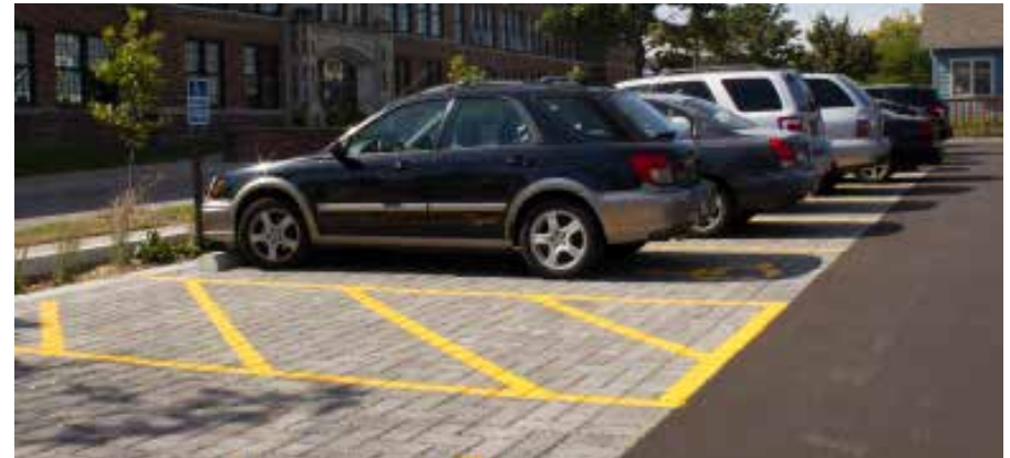
Example of a permeable pavements
